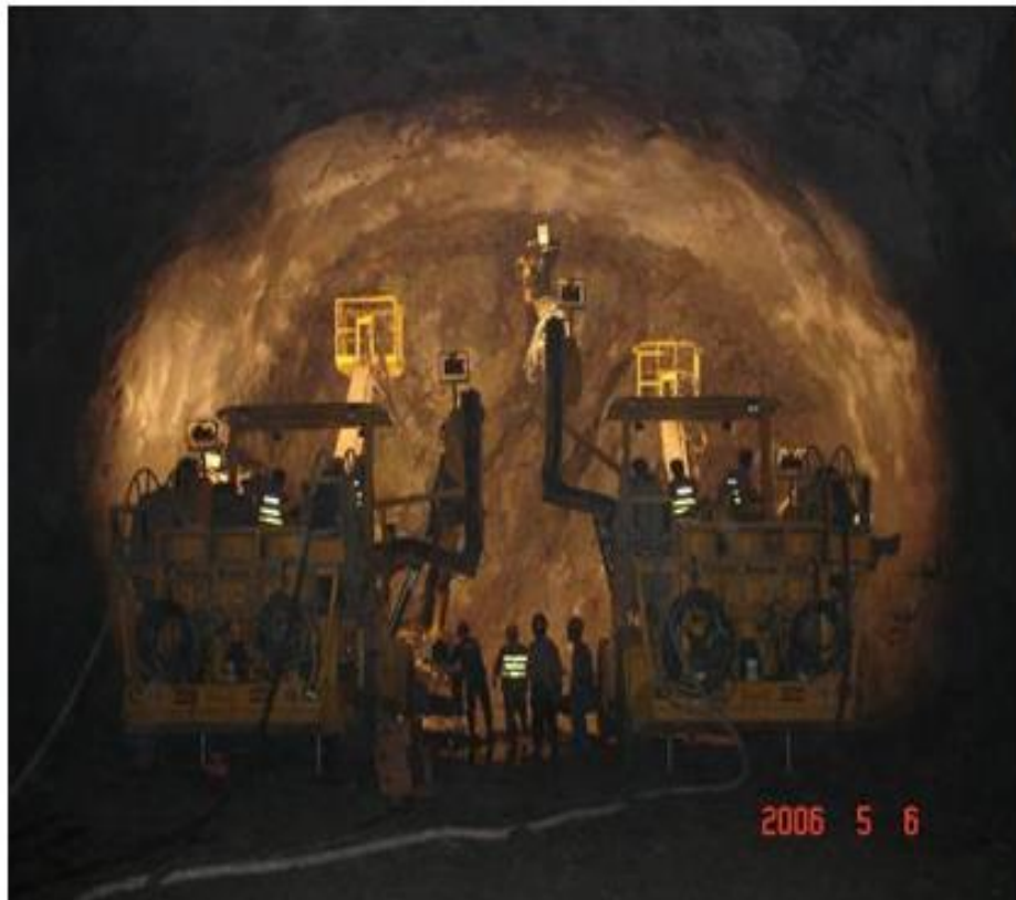
● 凿岩台车施工
