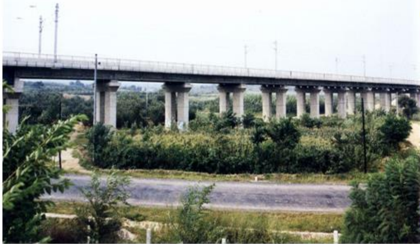
秦沈客专跨度16m四片式整体桥面T梁简支梁
